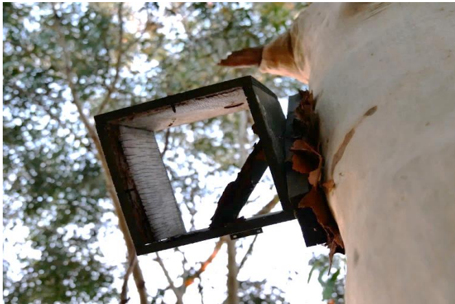
The lid and bottom of this possum nest box need to be replaced, and other maintenance may be required, for it to be returned to a condition suitable for use (Photo: Fern Hames)
